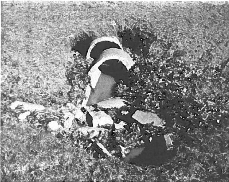
Aging, Failing Storm Drains
