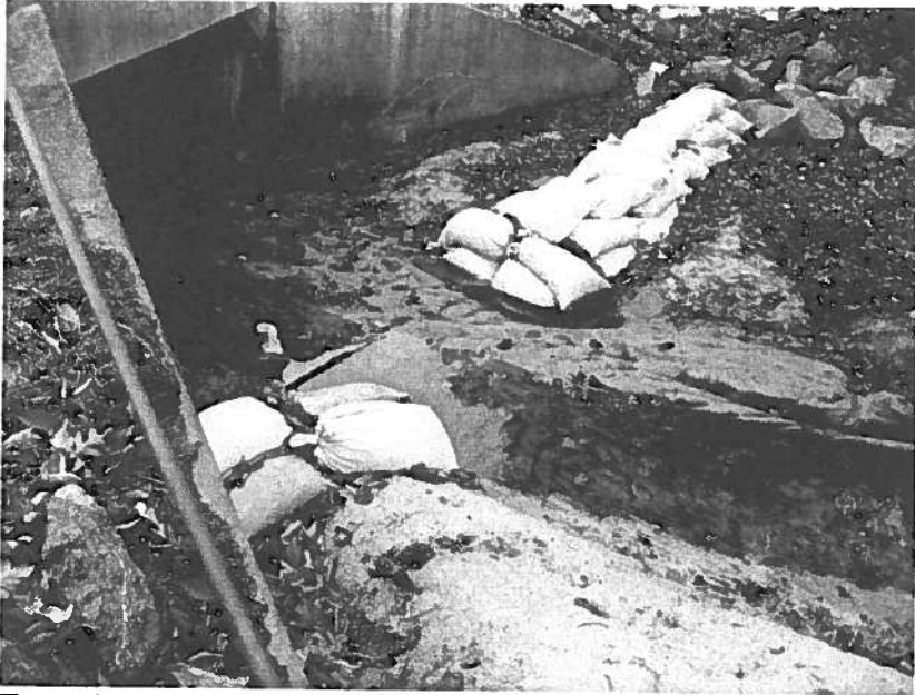
Excessive Erosion from Uncontrolled Runoff
